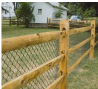
3- RAIL PINE with chain-link wire backing
