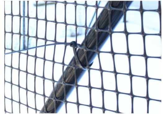
ZIP TIED TO POSTS
