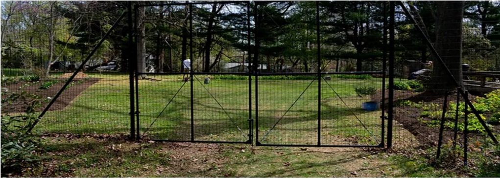
DOUBLE GATES FOR VEHICLE ACCESS
