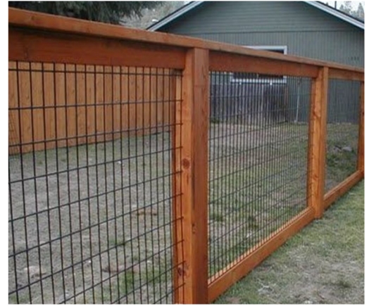
WOOD FRAMED, 2" x 3.5" WIRE WELD to meet CT minimum pool code
