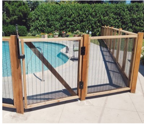
WOOD FRAMED WITH TIGHT WIRE WELD with tight spacing for animal abatement and pool
