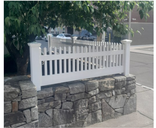
DRIVEWAY WALL & VINLY TOPPER in Victorian picketing
