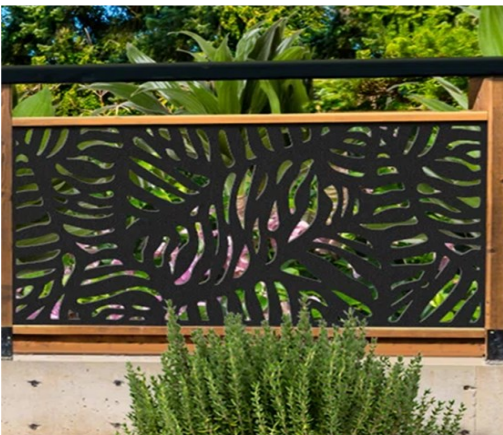
FRAMED VENEER TOPPER on poured concrete wall
