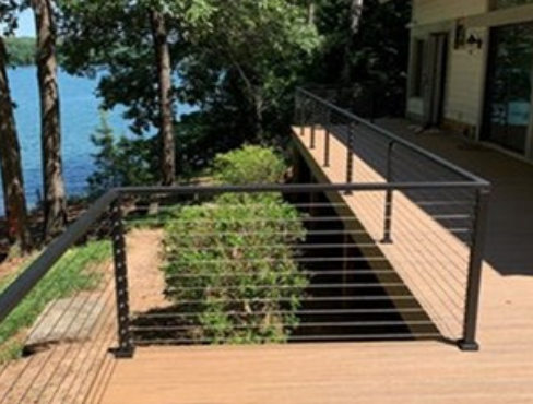
METAL POST AND CABLE with cable railing strung at 4" apart
