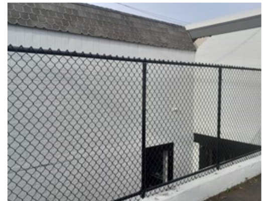
BLACK COMMERCIAL CHAINLINK for safety against drop off a top 1.0' retaining wall
