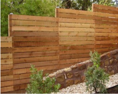
STEPPED WOOD ALONG RETAINING WALL in cedar with 4" x 4" posts
